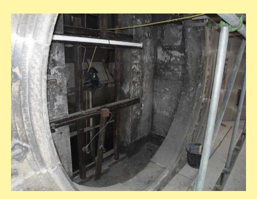
Deteriorated masonry joints and stone features are being replaced. The high-level scaffolding has enabled us to photograph some of the good quality stone carving, particularly of faces.
